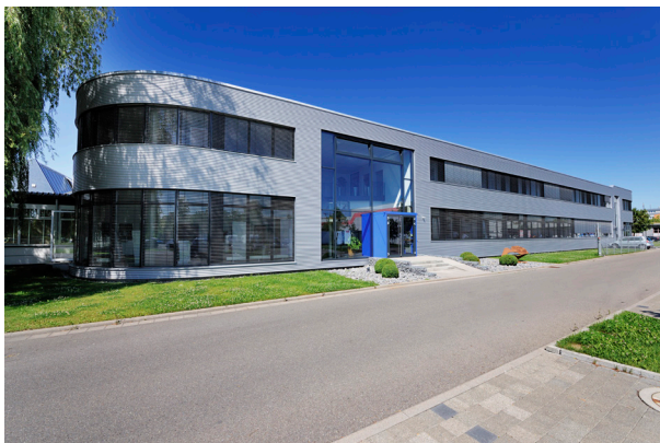
Figure 1: BVS Blechtechnik in Böblingen, Germany
